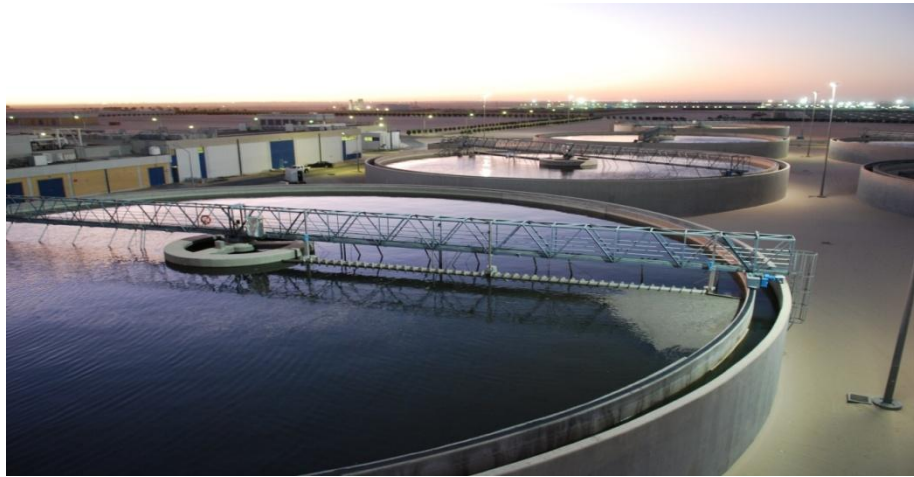
Figure 1: Wastewater Treatment Facility at Sulaibiya near Kuwait City
