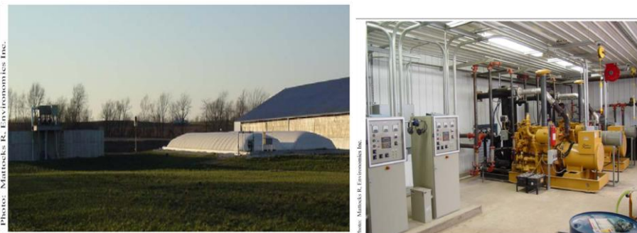
Figure 6. Plug-flow digesters and twin generators at New Horizons dairy
